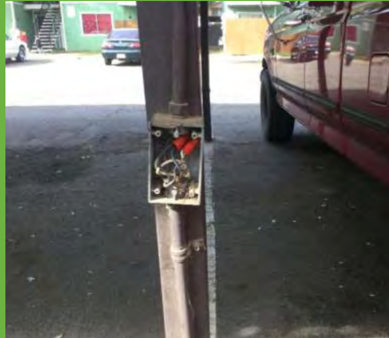
Exposed Wiring
